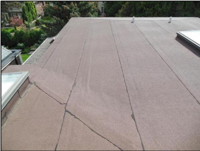
3. Modified bitumen membrane
