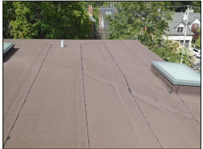
4. Modified bitumen membrane
