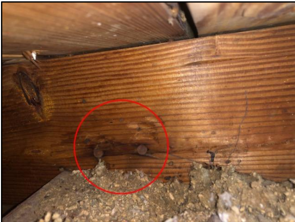
Roof to Wall Attachment
