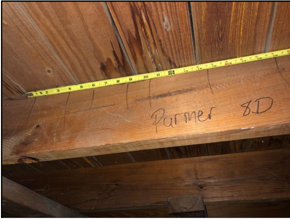
Roof Sheathing Nail Spacing Dimensional Lumber 1/2" thick with at least one nail per board
