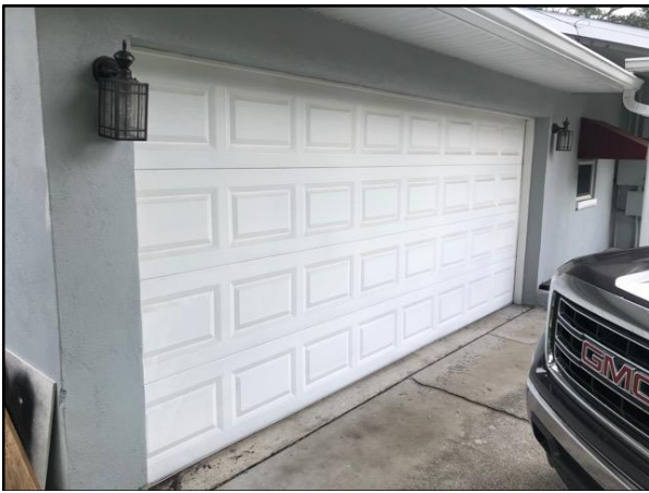
Garage Door Label No labels found rating garage door for wind or impact protection.
