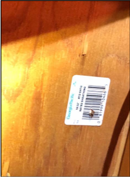
Roof Plywood Thickness
