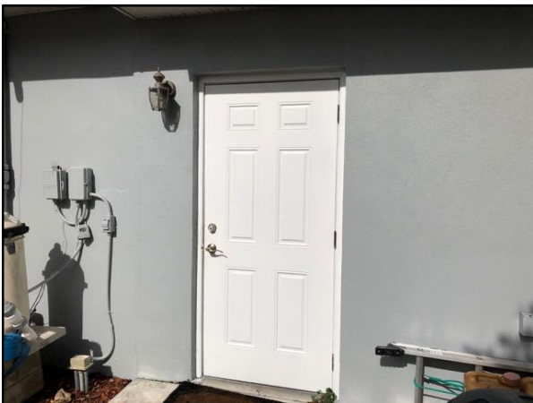
Front door is not impact rated and no labels are present. Both the Inner and Rear garage man doors are metal clad and appear to meet wind borne debris protection but no labels are present to confirm.
