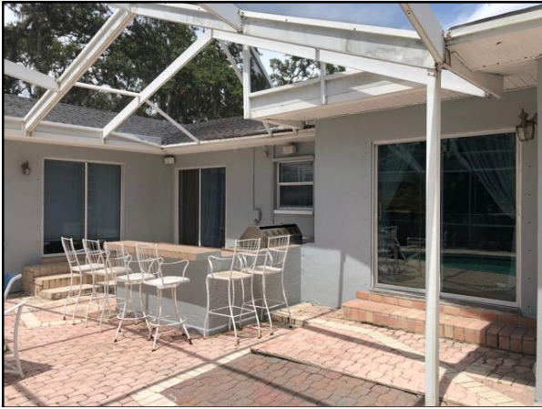
Sliding glass doors not rated for impact
