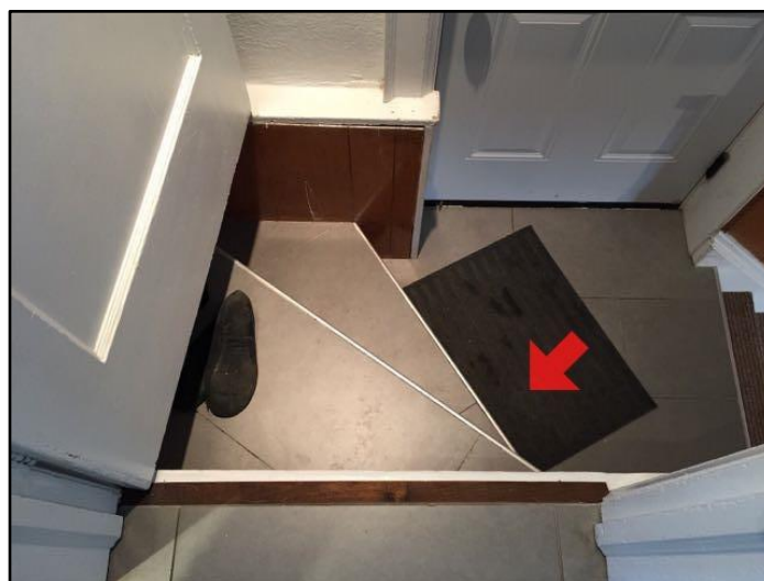
Width too small on curved treads
