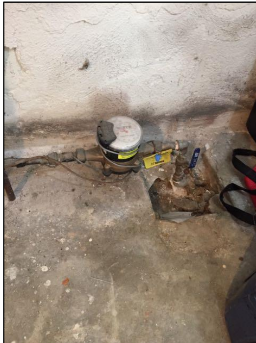
Front of the basement
