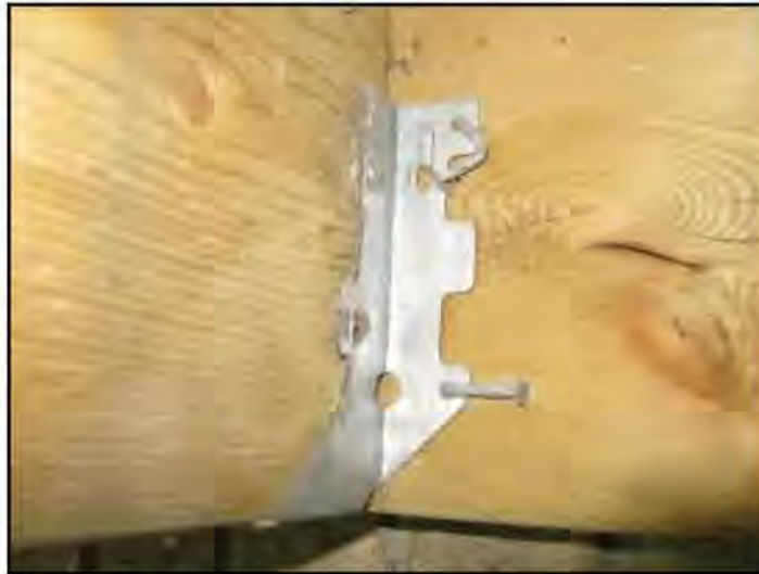
Poor end bearing, joist hanger connections
