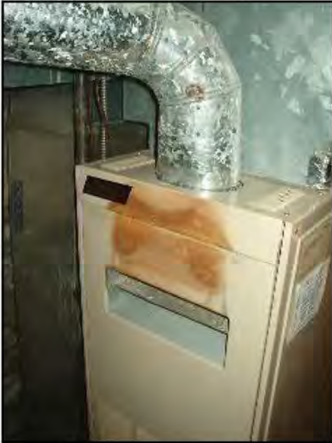
Draft hood spillage or backdraft
