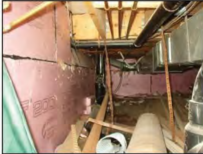
Exposed combustible insulation
