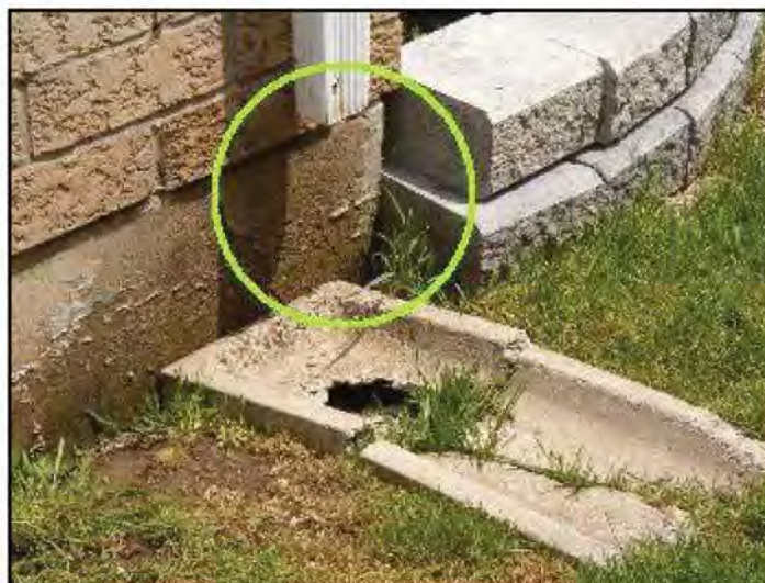
Downspouts discharge too close to building
