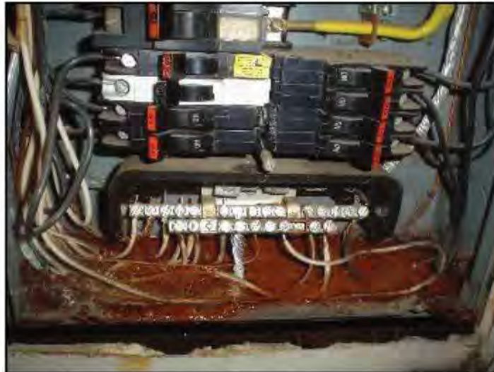
Water and rust in bottom of panel
