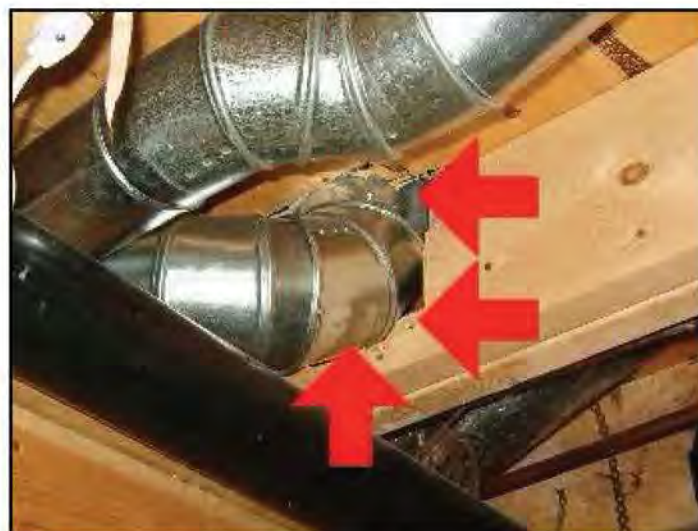
Joists are notched and weakened
