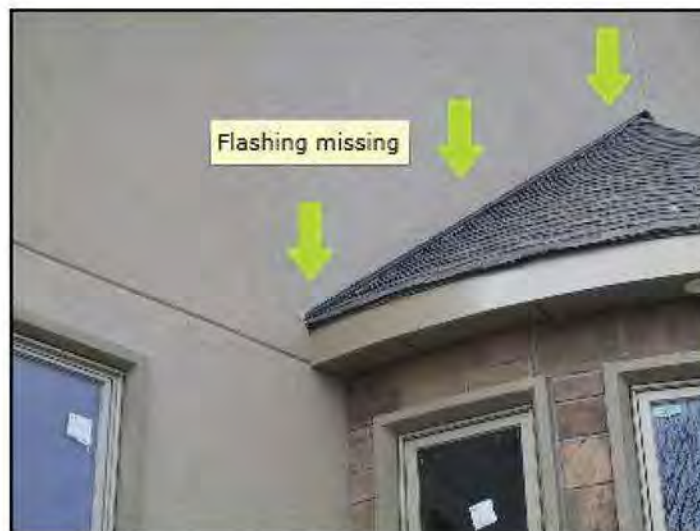
No kickout flashing at roof/sidewall junction
