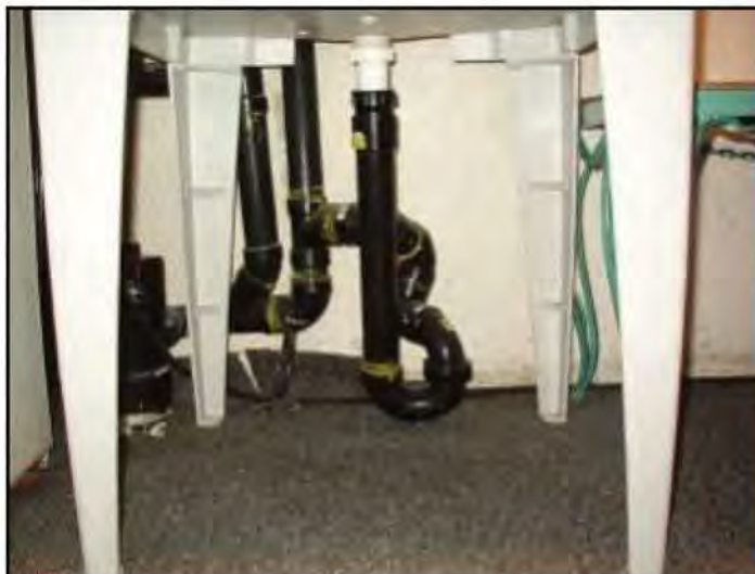
Poor trap arrangement
