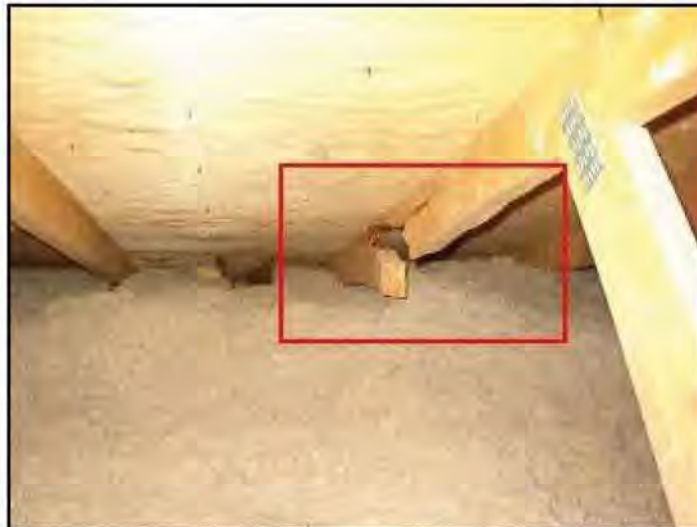
Top chord of truss is split
