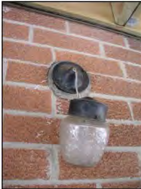
Light fixture is not well secured
